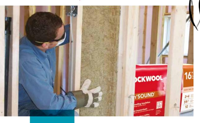
ROCKWOOL Safe'n'Sound® is a stone wool insulation for use in interior partitions of residential wood and steel stud construction where superior fire resistance and acoustical performance are required.
